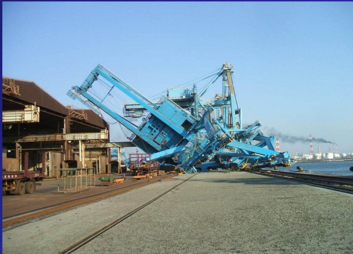
Crane that collapsed by large vessel
