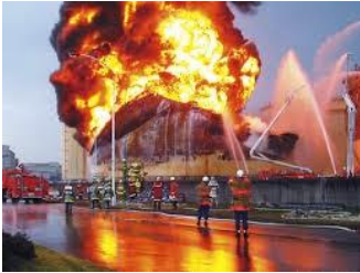
Tank fire caused by large earthquake (28 Sep., 2003, Hokkaido, Japan)
