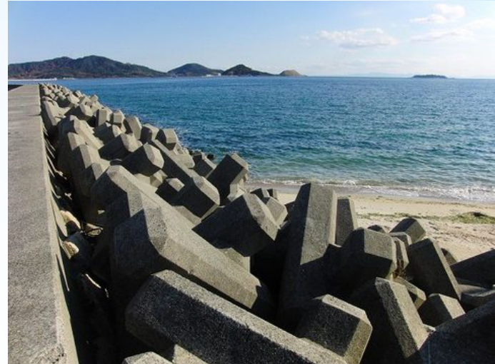
Embankment by tetrapods
