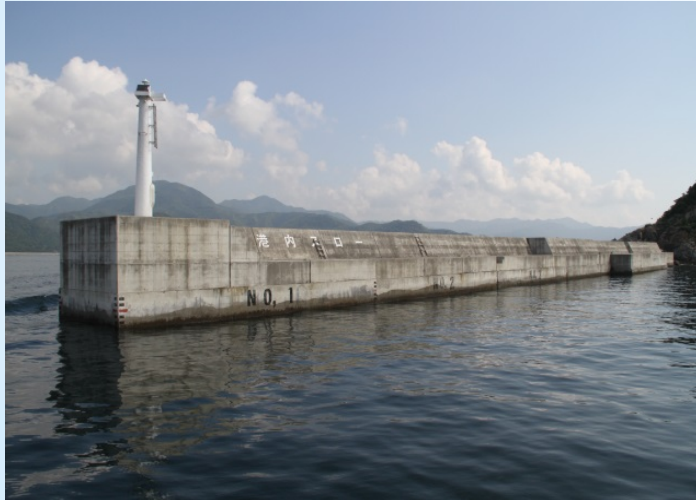
Seawall by concrete
