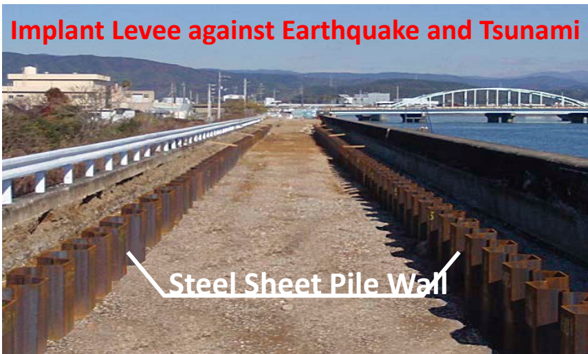
Protection of Coastal Dike by Steel Sheet Pile
