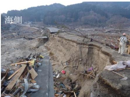
Photo 2 Eroded highway bank
