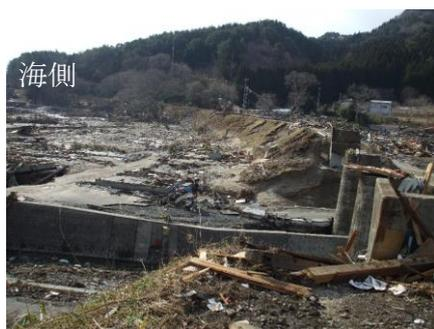
Photo 3 Eroded railway bank
