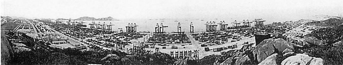
Figure 5: Yanshan Deep Water Container Terminal ( http://en.wikipedia.org/wiki/Yangshan_Port ).
